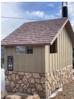
CXT Vault Toilet
